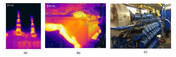
Figure 18: (a) The thermal image of the engine in operation mode. (b) The thermal image of the engine in standby mode. (c) Normal image of the engine.
