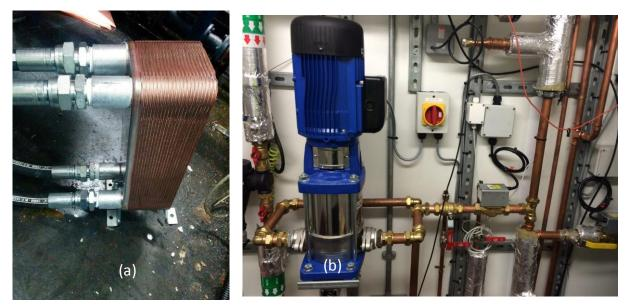
Figure 19: (a) Plate heat exchanger on the engine side to transfer and recovery heat. (b) Circulation pump to circulate heat to the engine.
