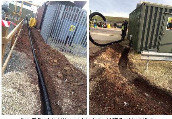
Figure 20: Pipes being laid to convey hot water from (a) GSHP container (b) Engine
