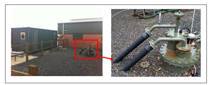
Figure 5: Mine water flow and return pipe.
