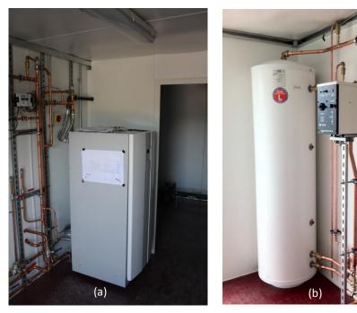
Figure 8: (a) Heat pump. (b) Buffer tank.
