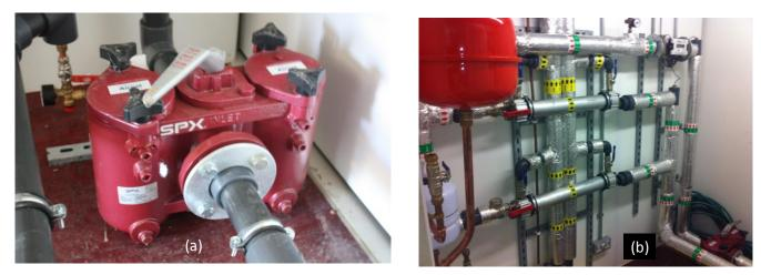
Figure 7: (a) Filter. (b) Heat exchanger.
